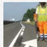
Applying PREMARK® is fast and simple because all you need is one person, a broom and a portable gas burner
